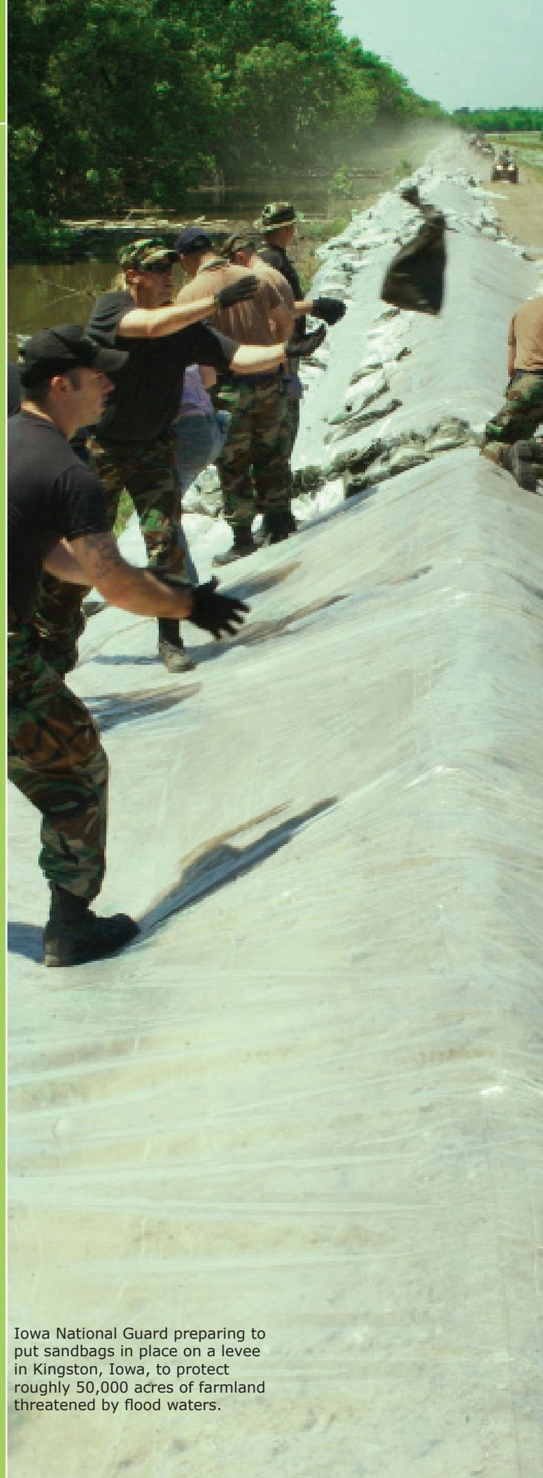
Iowa National Guard preparing to put sandbags in place on a levee in Kingston, Iowa, to protect roughly 50,000 acres of farmland threatened by flood waters.
